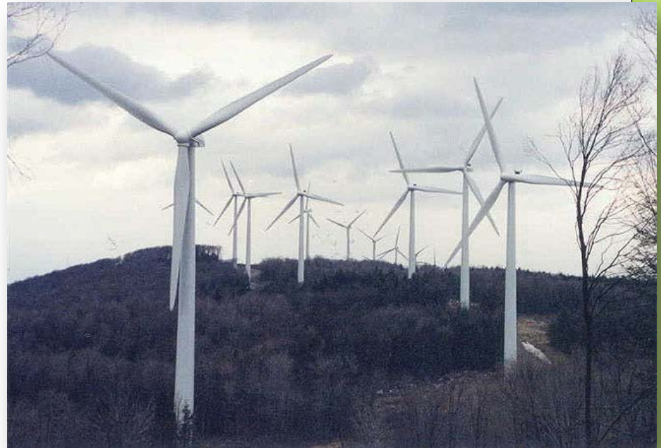
Mountaineer Wind Energy Center, WV www.communityenergy.com
