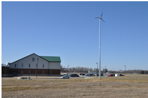
Figure 1: Skystream installed at Northumberland Middle/High School
